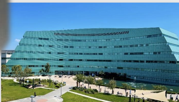
Kaiser Permanente Baldwin Park Medical Center, Baldwin Park, CA
